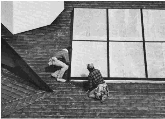
"New copper shingles can be installed easier than almost any other roofing method. Just snap two copper shingles together, and then put in two copper nails. No highly skilled craftsmen are needed," says the principal architect of this Denver home and member of the legendary Wright Foundation.
